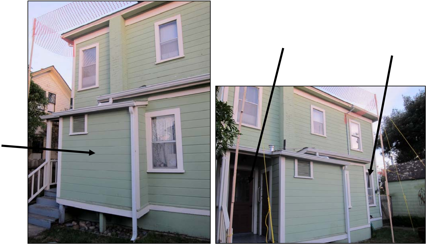
Figures 3 and 4. Two images of the rear (west) elevation. The left image looks northeast and shows the second rear addition with an arrow. The right image looks southeast and shows the circa-1901 entry porch to be removed (left arrow) and the window opening to be converted into a new rear entry (right arrow).
