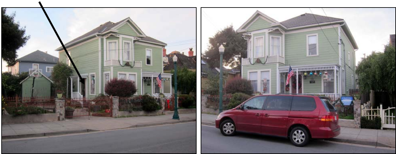
Figures 1 and 2. Left image shows the front (east) and side (south) elevations of the house as constructed circa-1901. The side entry porch is an addition possibly dating to the 1940s/1950s (arrow). The garage located to the south replaced an earlier garage by 1926. Right image shows the front, Forest Avenue elevation with Queen Anne-style design features and projecting second-story, clipped-bay window.
